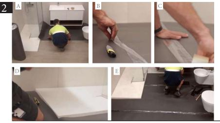
To install FAUS flooring on any surface, you should always use a comfort base that includes a plastic film with a moisture barrier ('underlay') In addition to its levelling function, it will also reduce the acoustic vibrations caused by footsteps and impacts.
