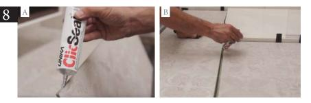
It is not necessary for general installations, but in areas with large and continuous water spills, it is recommended to apply our Clic Seal sealer. This should be applied to the tongue side of the click system.
