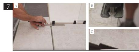
In areas where we cannot place the full plank, we measure and mark the space where the plank needs to be cut fit with a pencil, always ensuring to leave the appropriate expansion joint.
