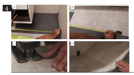
Insert the next plank at an angle. Follow the same procedure for the entire row. Mark and cut the last piece (a wood saw must be used).
