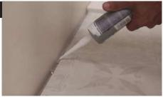
Once the profiles have been measured and cut, it is time to apply flexible silicone around the perimeter between the floor and the wall, as well as between the planks which forms the expansion joint. After completing this step, the aluminium profiles can be installed.
