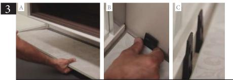
Start assembling the floor from the left corner. Place the first plank with the tongue (the edge with fewer mechanical components) towards the wall and insert expansion wedges between the wall and the plank. We recommend trimming the protrusion of the tongue to avoid issues with the expansion joints. Both the expansion joint, and other fixed elements, should be 10 - 12 mm wide.
