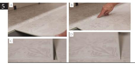
Start installing the second row according to the design pattern chosen. For example, for the design shown on the images, it should be cut to match the bevels indicated on each tile (approximately 50% of the plank from the previous row). In the case of a wood or stone design which allows it due to their structure, you can use the last piece from the previous row if it is longer than 40 cm.
