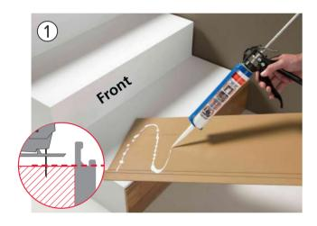
With a dry and levelled surface, cut the FAUS floor at the level of the risers (front) height, subtracting 80mm (size of the stair nose) and cut the tongue and groove of the 4 sides.
