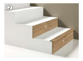
Once the front is glued, cut the stair nose profile to the size of the step, without sticking it.
