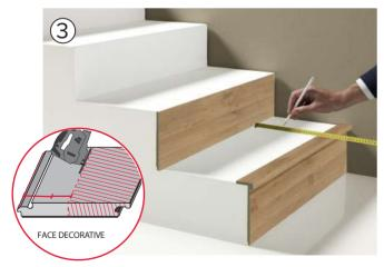
Measure the length of the step. Cut the piece of floor, leaving the decoration down. Transfer the measurement taken previously adding 2mm, counting from the male side. Then cut the piece of floor.
