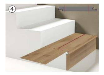
Measure the length of the step and and cut the plank at both sides to the measure, make sure to clean both the tongue and the groove transversal.
