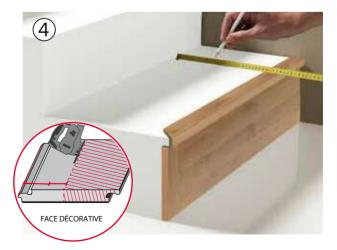
Provisionally, place the stair nose and measure the distance (riser) from the front to the profile. Next, cut the plank facing the decorative side down. Note that you should add 2mm to the previously measured distance, counting from the side of the tongue.
